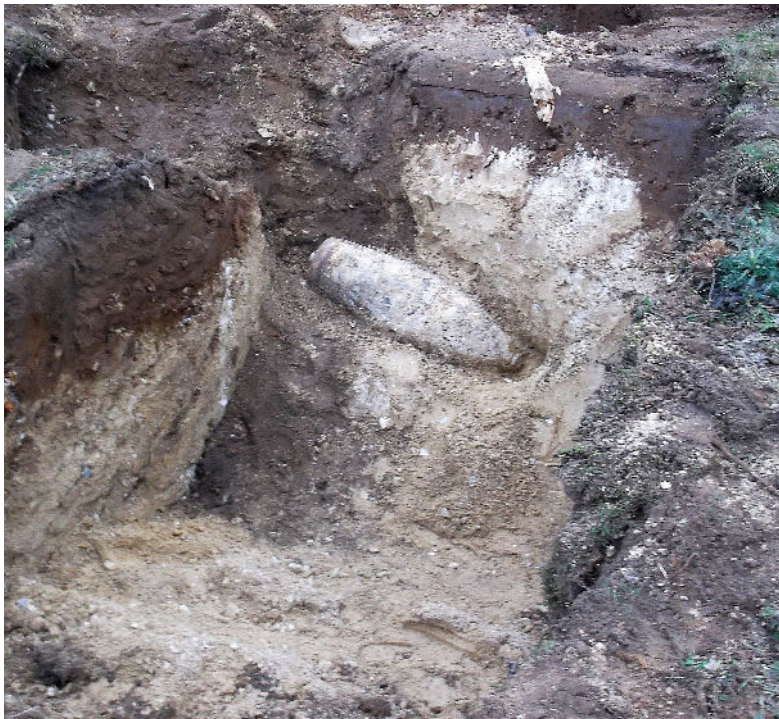
Image showing a British 500lb HE unexploded bomb during excavation operations at a site in Thetford, Norfolk.
